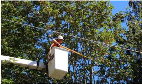
Tree limbs that occasionally brush against a service line won't damage it. But a limb or trunk that is pushing a service line out of its normal path should be trimmed or removed.
